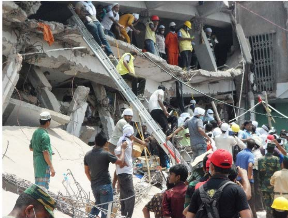
Figure 2: Rana Plaza building collapse
